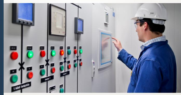
The control system of IntelliStore™ solution is an individually configured ENTSO-E compatible VPP system, which allows to control the system from the built-in touchscreen, from anywhere around the globe through the internet and the remote control system, just as well as from the headquarters of the TSO/DSO. At the same time, the system is capable to act automatically, following and equalizing pre-entered schedules.
